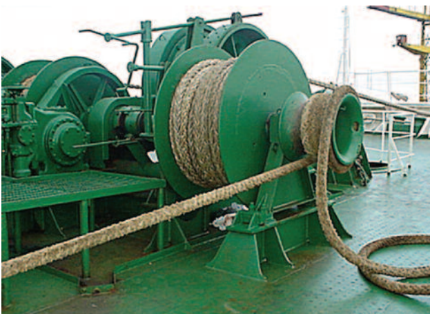
Well painted but poorly highlighted mooring station
