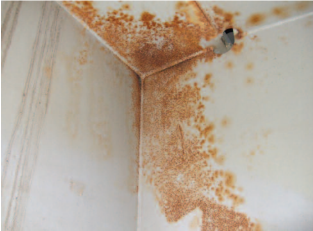
Scattered corrosion
