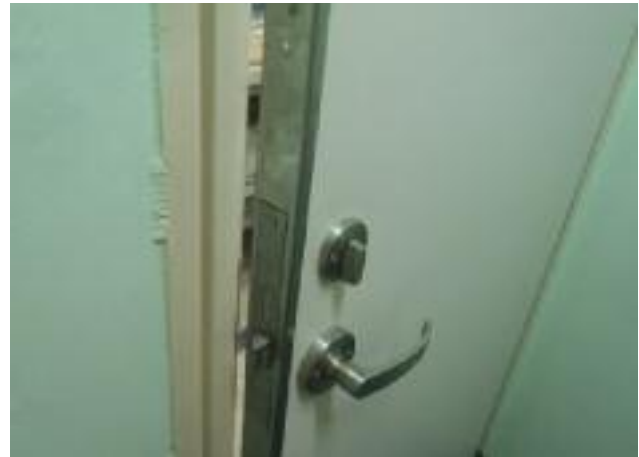
Fire door failing to close
