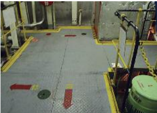
Arrows leading away from exit door
