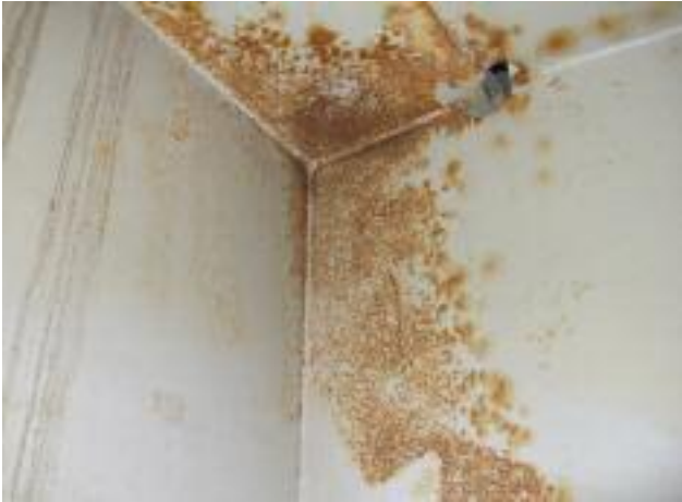
Scattered corrosion
