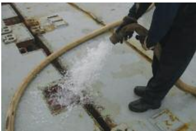
Filling up of interpanel void space with water from a fire hose without a nozzle
