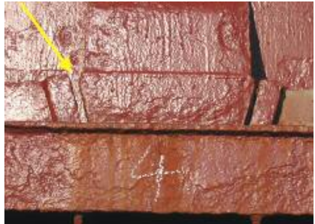
Excessive wear on locator
