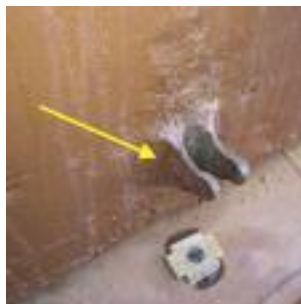
Corrosion and diminution of a quick acting cleat crutch and thinned down snugs
