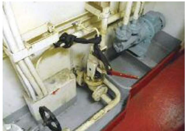
Quick closing valve held open with a stop
