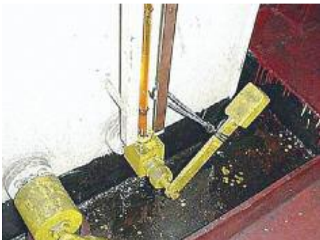
Self-closing gauge glass held open with string
