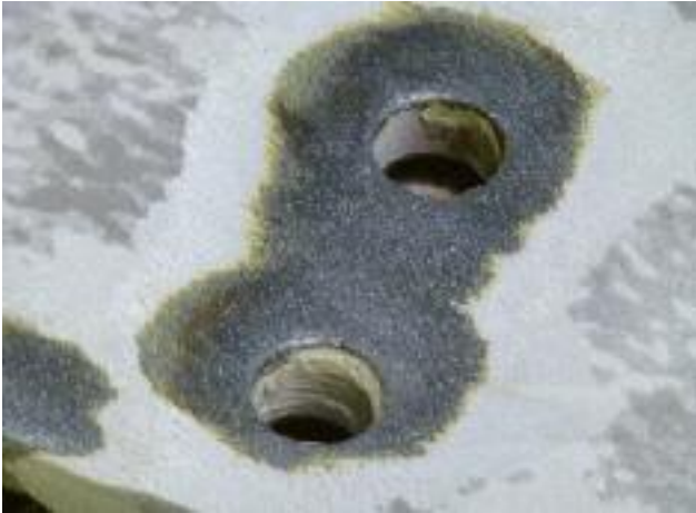
Repair area with profiled surface ready for painting
