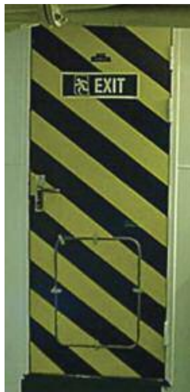
Well marked door
