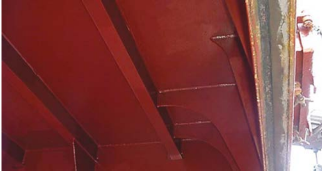
Figure 1.7: Hatch undersides and rubber packing.
