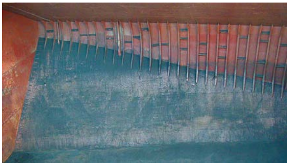
Figure 1.15: Tank showing previous cargo residue.
