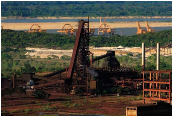
Figure 10.1: Direct reduction plant which reduces iron ore to produce direct reduced iron.
