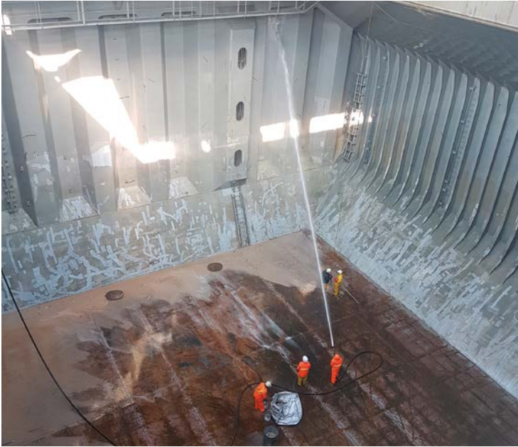
Figure 17.1: Crew undertaking hold preparation.
