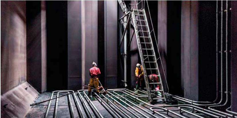
Figure 18.5: Tank cleaning in progress.
