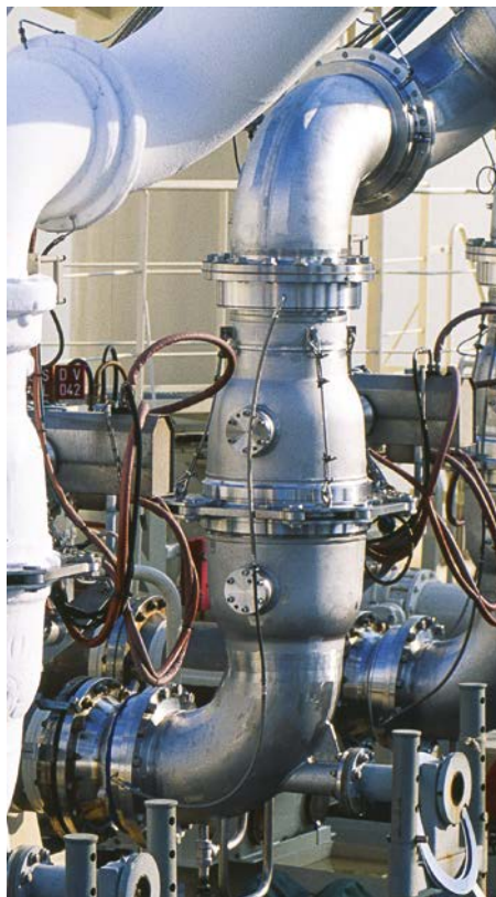
Figure 23.8: MLA connection to manifold, showing double ball valve safety release.
