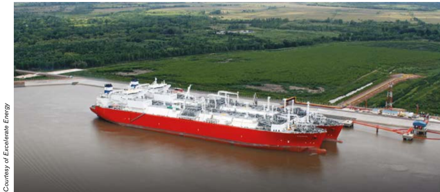
Figure 24.10: Transshipment of LNG to an FSRU on a regas berth.
