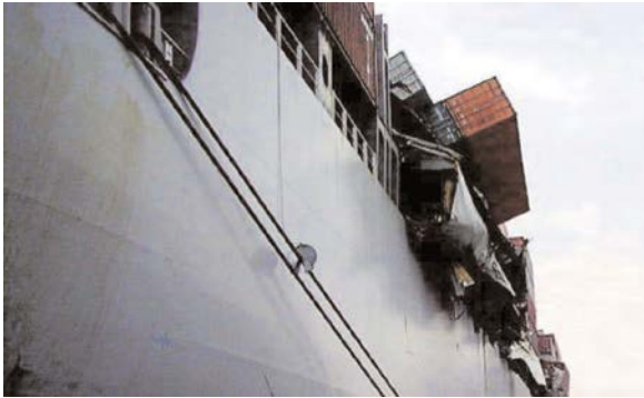
Figure 41.14: Collapsed container stacks as a result of bad stowage.
