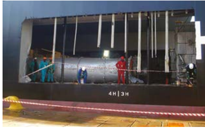
Figure 45.19: When sea fastenings fail under excessive vessel motions, the violent motion of large, heavy project cargoes can cause extensive damage to the vessel structure. Side-shell plating (in way of cargo holds), deck structures and hatch covers are particularly vulnerable to damage. The repairs can cause extensive delays.
