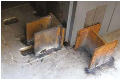
Figure 45.32: 'Hard' sea fastenings.
