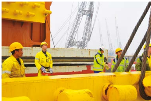
Figure 45.11: A clear understanding of each party's responsibilities and good teamwork is key to the success of project cargo transportation.
