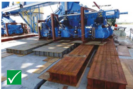
Figure 45.20: Load-spreading 'mats' to protect the structure of the vessel.
