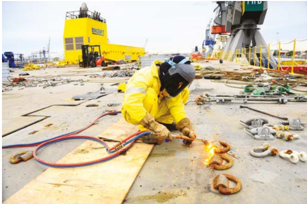
Figure 45.21: Adding securing points to the deck of a heavy-lift vessel.
