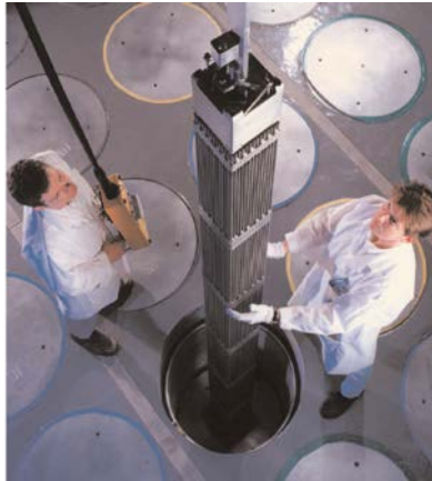
Figure 49.4: Nuclear fuel assembly being loaded into nuclear power plant.
