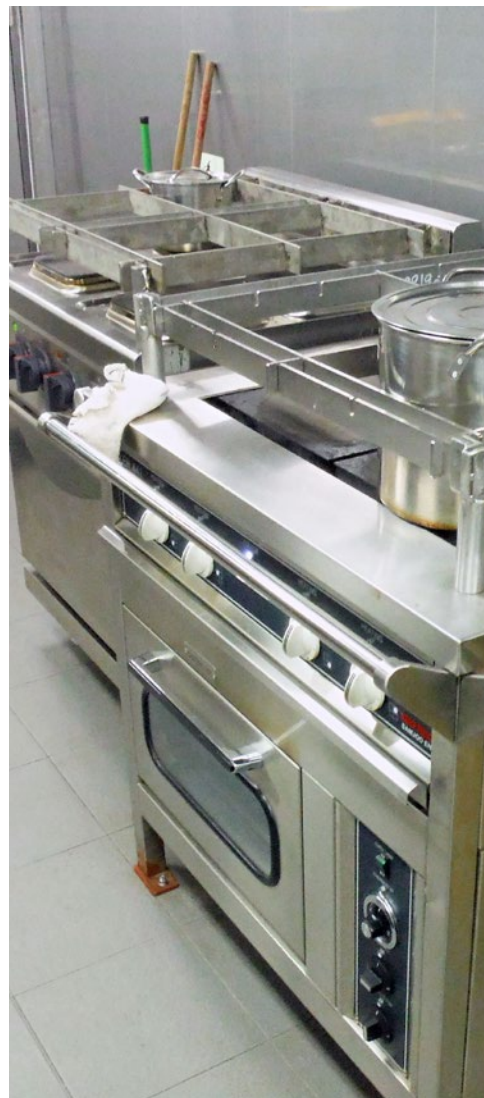
✓ Galley stove fitted with storm rails and grab bar.
