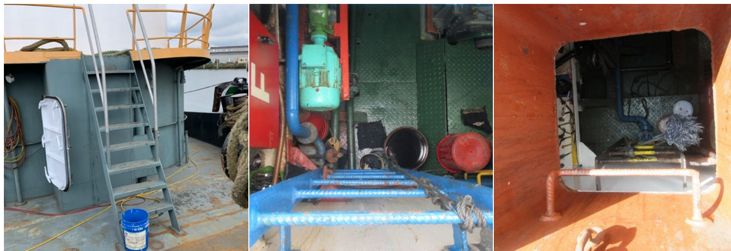
X Trip hazards at the top and bottom of ladders.
