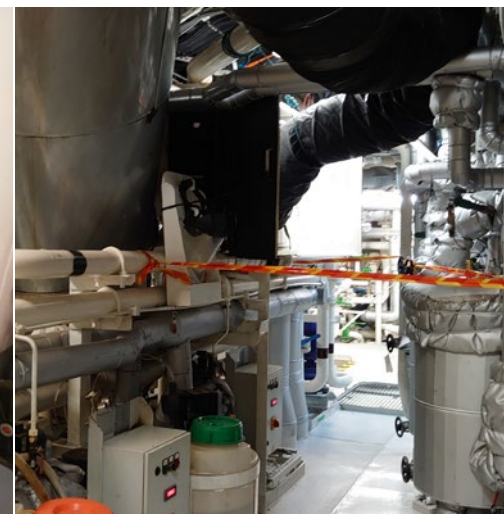
✓ Stanchions and chains/bars readily available at low level hatches, and tape used in other areas to control access
