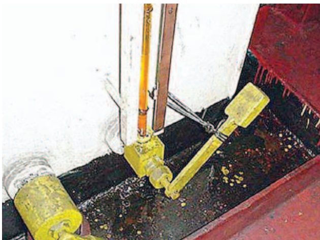
Self-closing gauge glass held open with string
