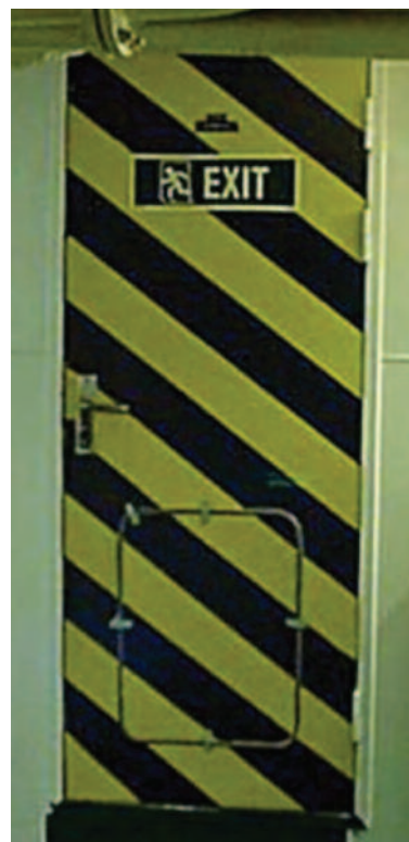
Well marked door
