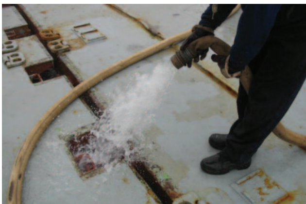
Filling up of interpanel void space with water from a fire hose without a nozzle
