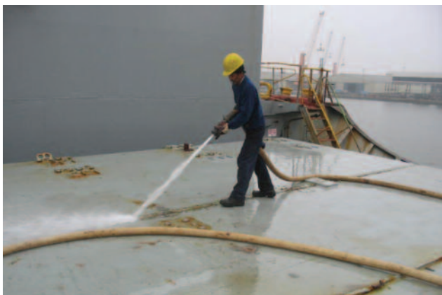
Strong jet of water being applied to the cross joint
