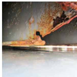
Cracks and corrosion will affect the panel's structural integrity
