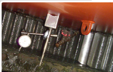
Measuring wear of the slew bearing
